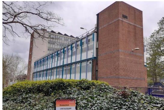
Figure 2. North entrance, looking east along Cope Street
